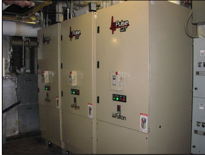
Figure 15- Installation of New Energy Efficient Boilers at CCI
