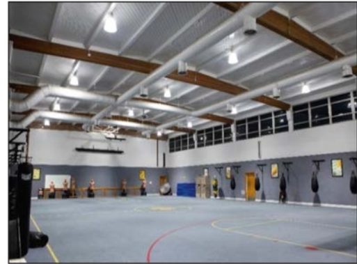
Figure 17- Energy Efficient LED Fixtures
