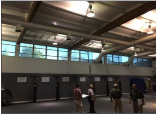
Figure 16- High Pressure Sodium Fixtures
