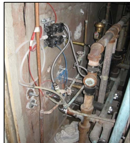
Figure 31- Flushometers at CMF
